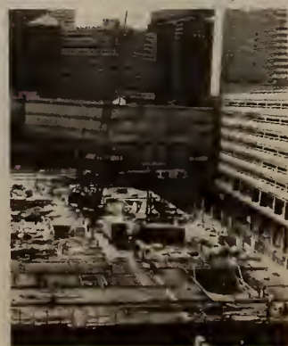
Back Bay Station lobby deck under construction.
